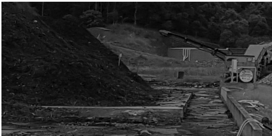
Figure 8. Under-bed compost aeration system at Lismore. Photograph: Peter Booth
